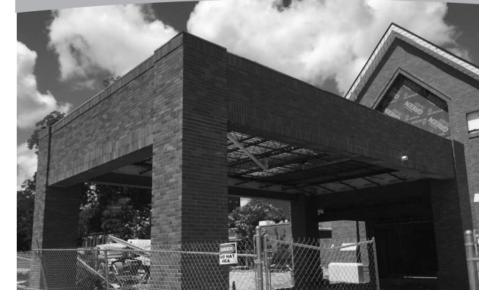
New covered entry
